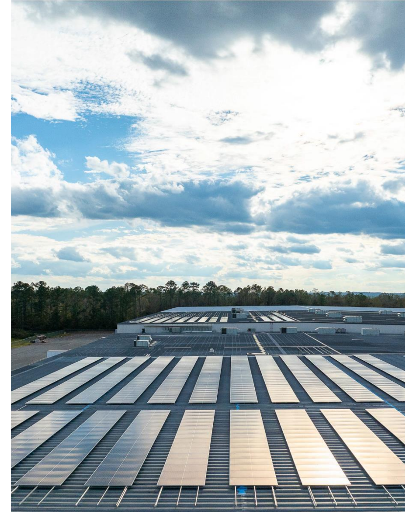
Tumi Vidalia Headquarters Solar Panel Installation
